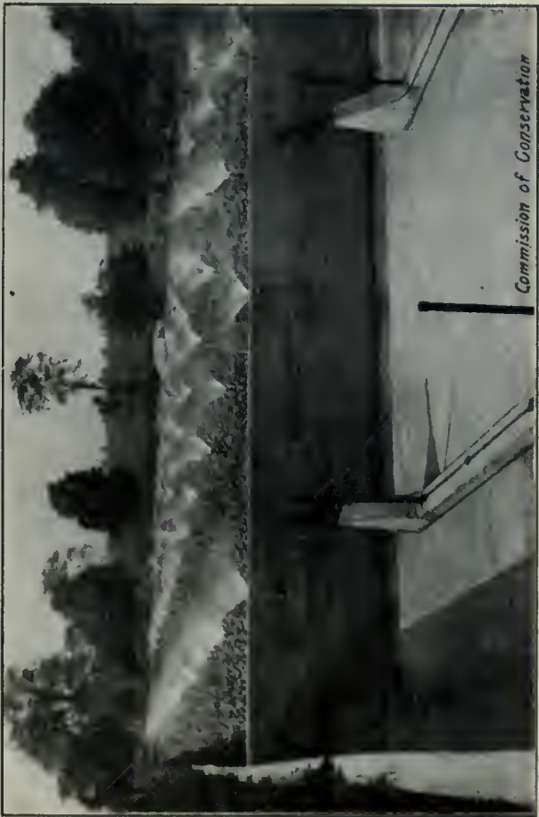
Stratford Sewage Disposal Works—Sprinkling Filters (Summer View).
